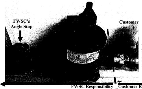
Customer is required to install a personal cut off valve about two feet after the meter.
