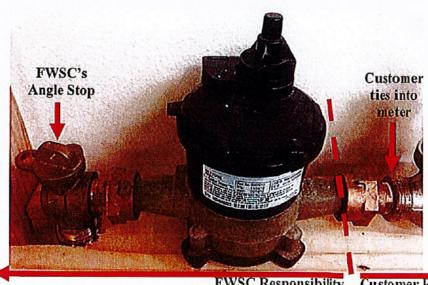
Customer is required to install a personal cut off valve about two feet after the meter.
